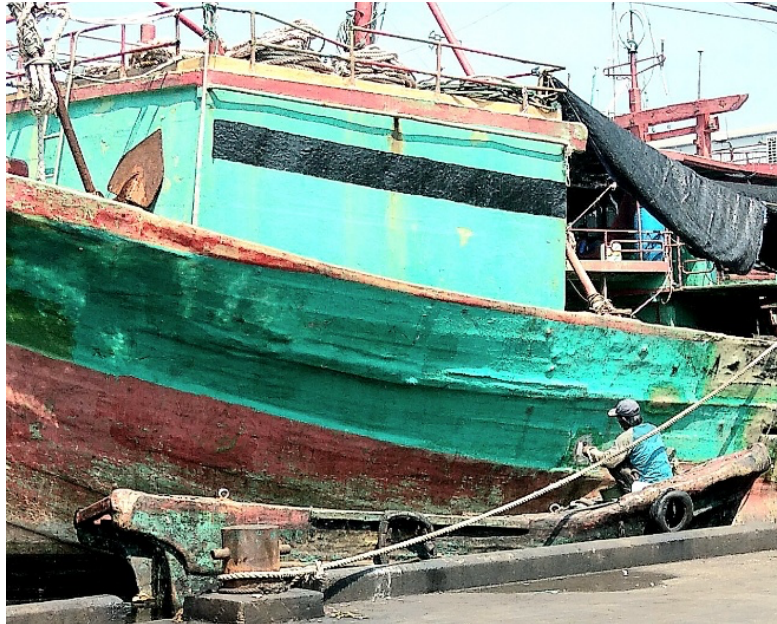
Figure 4 Workshop worker painting vessel hull at pier
