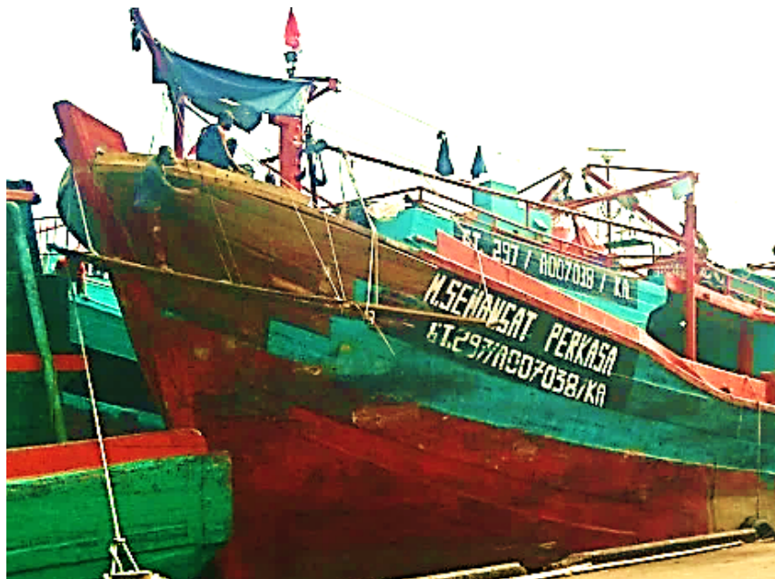
Figure 3 Workshop worker doing hull repair at pier
