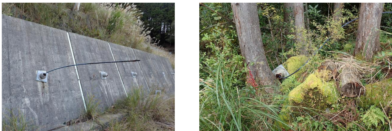
Figure 7. Anchor popping out
