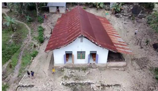
Sumber: Survei drone 2025
