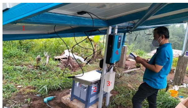
Keterangan: 1 = Solar panel; 2= Baterai; 3 = MCB dan kotak MCB; 4 = Inverter
