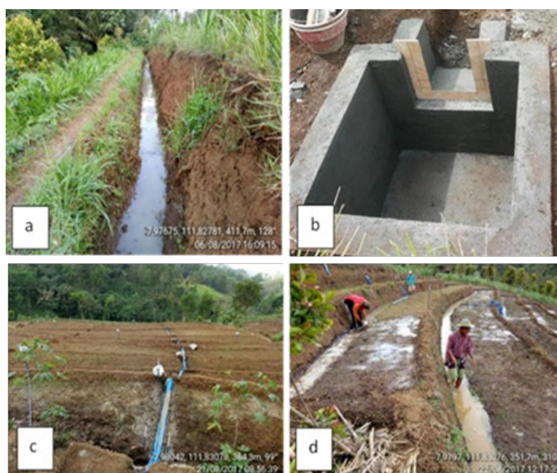
Figure 3. Water distribution through channels and the water level setting in the weir.
