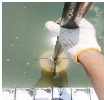
Figure 8 Waterproof test on portable underwater lamp construction.
