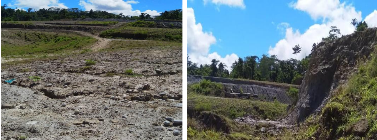
Figure 5 The planned upstream watershed for the built-up area has been partially leveled (left). Some of the lands is still steep and made like a ladder (right)
