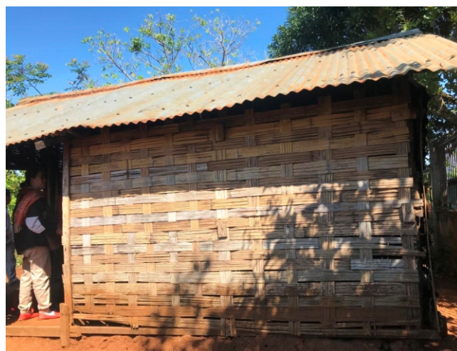
Figure 3 An IM house made of bamboo and wood in the buffer zone of BGMNP.
