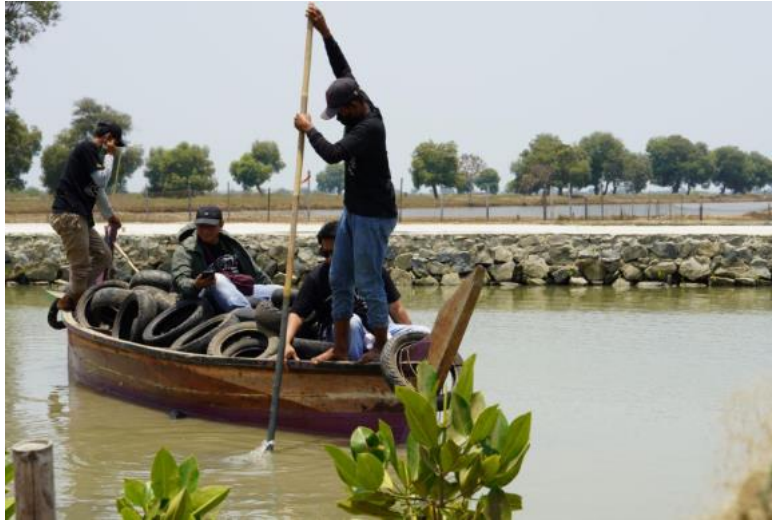
Figure 8. CSR support from Planet Ban for the implementation of APO (waste-tire wave breakers) coastal protection structures in Tanjung Pakis Village, Karawang Regency, Indonesia
