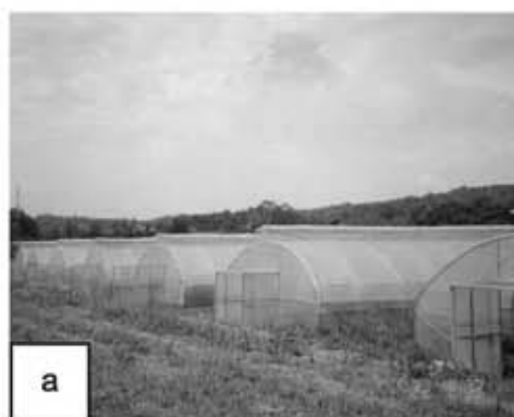
Figure 2. Naturally ventilated tropical greenhouse structures. (a) Single-span greenhouse (b) Quadruple-span greenhouse. "Reprinted from Journal of Tropical Agriculture and Food Science . (in press) Reference No.17/2006, Kamaruddin, R. and Faisal Mohammed Seif Al-Shamiry. Natural Ventilation by Stack Effect in Multi-Span Tropical Greenhouse Structures, with permission from the author."
