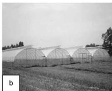
Figure 2. Naturally ventilated tropical greenhouse structures. (a) Single-span greenhouse (b) Quadruple-span greenhouse. "Reprinted from Journal of Tropical Agriculture and Food Science . (in press) Reference No.17/2006, Kamaruddin, R. and Faisal Mohammed Seif Al-Shamiry. Natural Ventilation by Stack Effect in Multi-Span Tropical Greenhouse Structures, with permission from the author."
